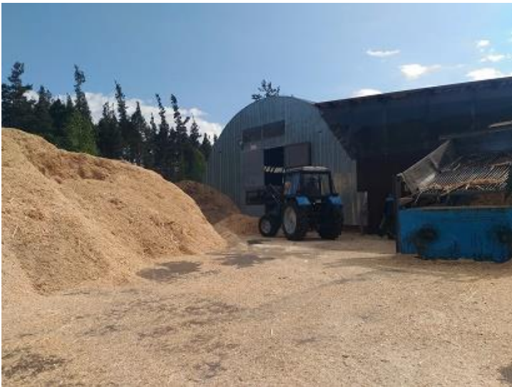
- - Overview of biomass manufacturing plant
